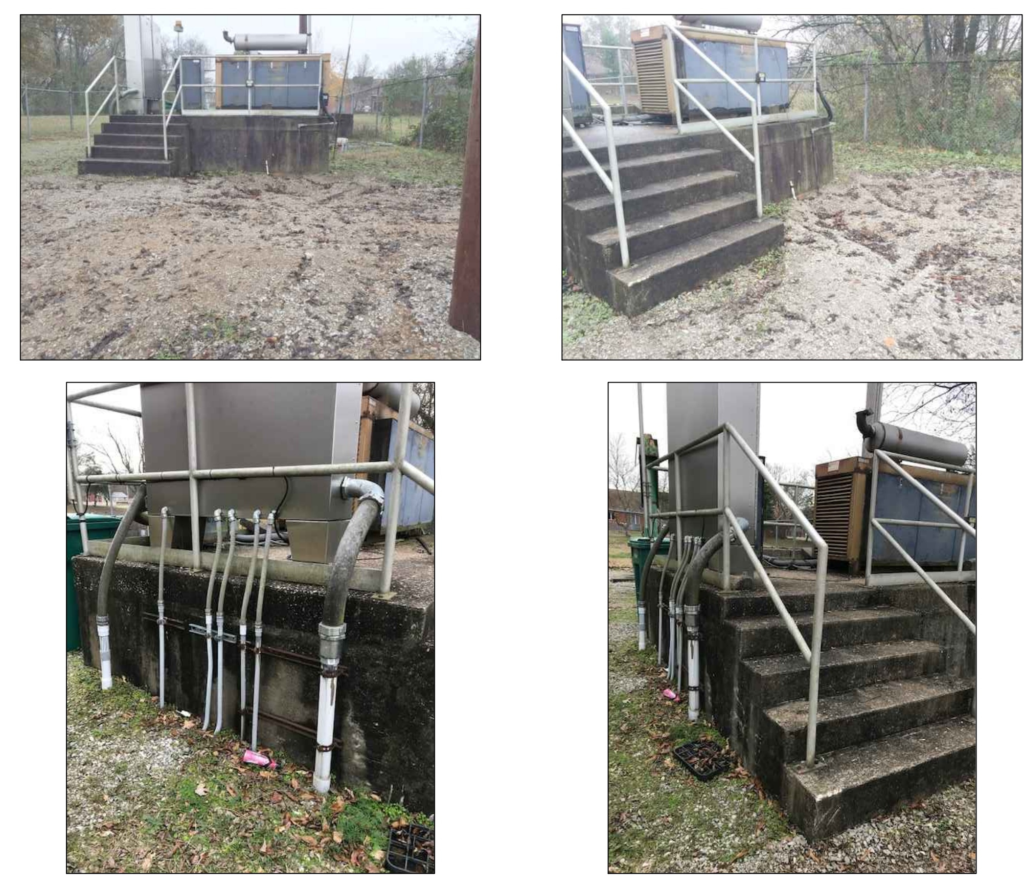
GENERATOR PAD: EXISTING SITE PHOTOS SCALE: NONE
