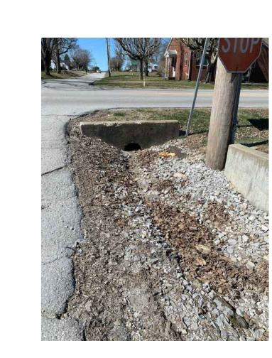
PROPOSED 'POUR-IN-PLACE' RETRO-FIT FOR CURB BOX INLET (TYPE F) SIMILAR TO KYTC DWG. RDB-320-06 (EX. 18" CULV); ~STATION 22+ {EX. INV. = ~642.8'; GRATE TOP = ~644.8'; VERIF`
