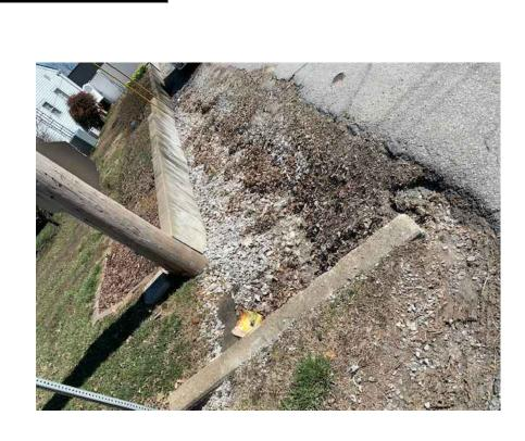
PROPOSED 'POUR-IN-PLACE' JUNCTION BOX (SIMILAR TO RDX-001-06) & HEADWAL (SIMILAR TO RDH-005-02; STATION  $\sim$ 30+63 {INV. = 653.5'; TOP OF SIDEWALK = ROAD EDGE & TOP OF NEW HEADWALL =  $\sim$ 655.7}
